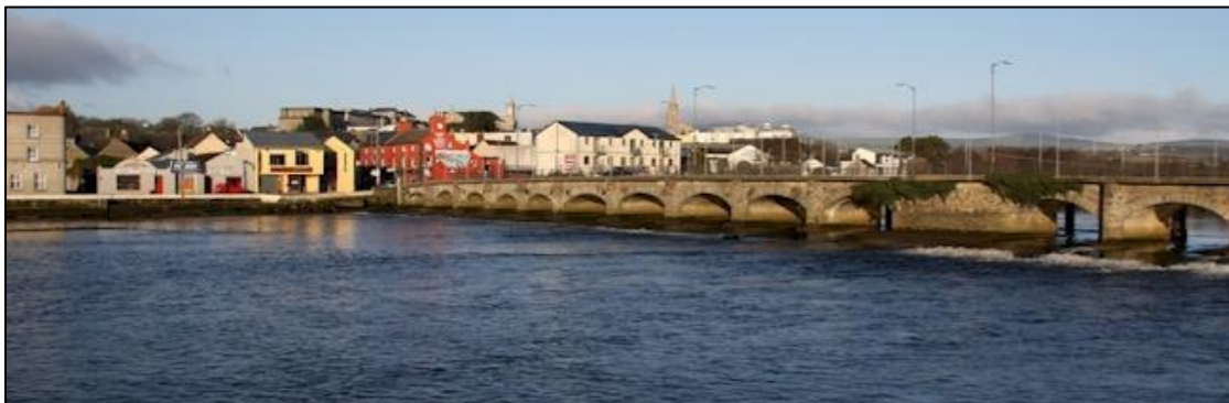
Figure 5-5: The 19 Arches Bridge
